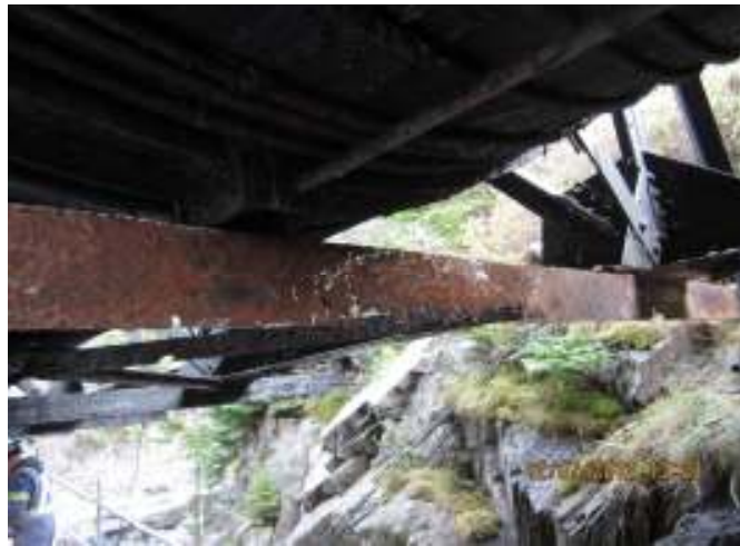
Figure 3 – Corrosion of Trestle Members
